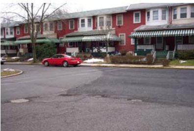
Juniata Terrace Borough street paving project.
