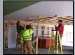
As of January 4, 2011, the exterior walls have been framed and sheeted with metal. The exterior doors have been installed and drywall has been hung on the ceiling where enclosed. A portion of the electrical service equipment has been donated by Lepley Electric of Lewistown. The final electrical service will be installed soon. Granville Township employees are completing the work this winter and spring.
