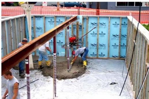
On July 10, 2006, contractor Tony Grose poured the concrete floors of both units of the duplex. A skilled Habitat for Humanity crew is currently framing the structure, which is anticipated to be under roof by late August 2006.
